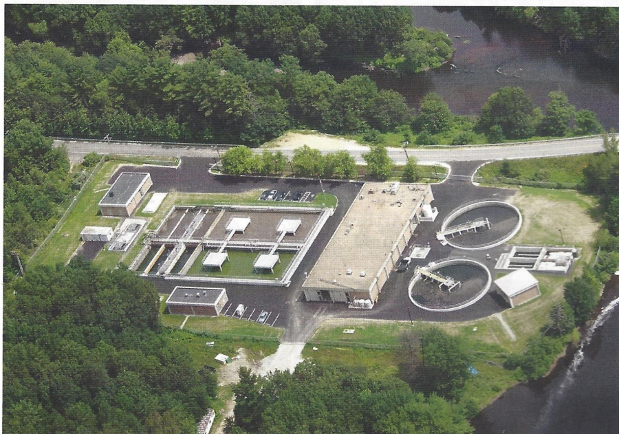
The Somersworth, N.H., water resource recovery facility treats wastewater for 11,800 residents. City of Somersworth, New Hampshire
